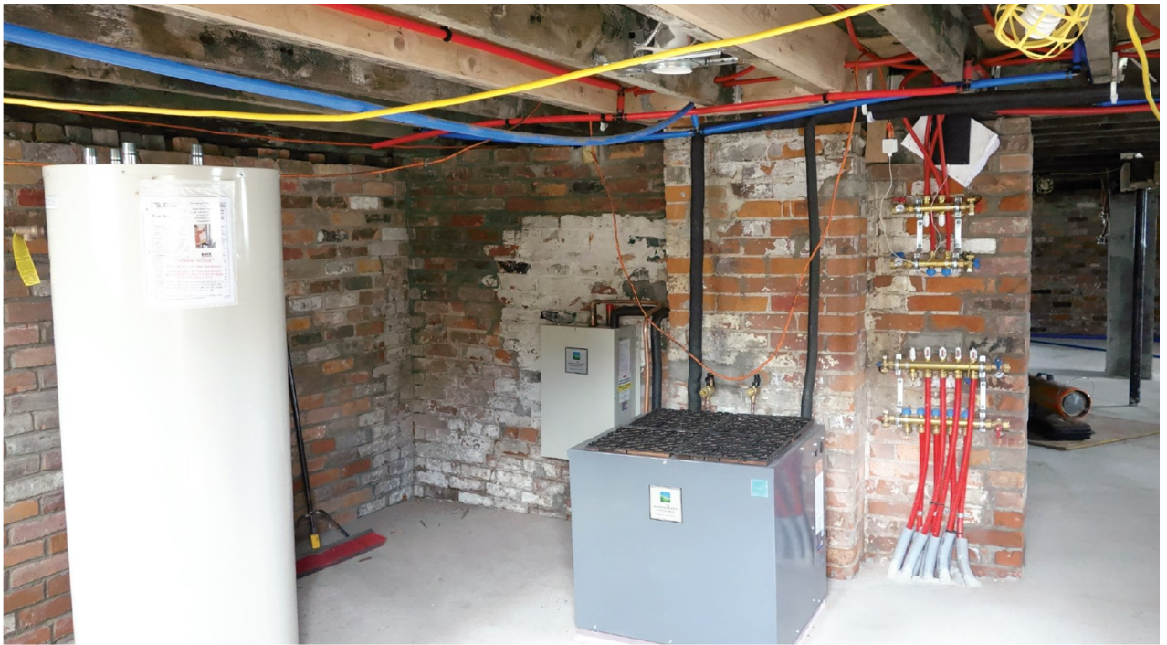
Direct-exchange systems are split systems by design, easily enabling forced air, radiant floor, and hot water assist technologies.
