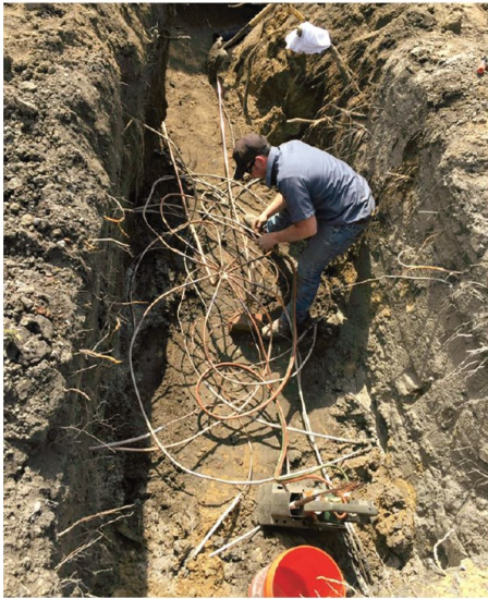
The high thermal conductivity of copper enables a small system footprint. Photo provided by: EarthLinked Technologies, Inc.
