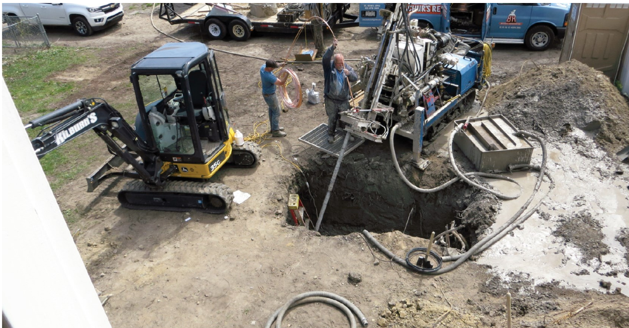
Drilling and loop installation activities took place over the course of a single work day. Photo provided by: EarthLinked Technologies, Inc.
