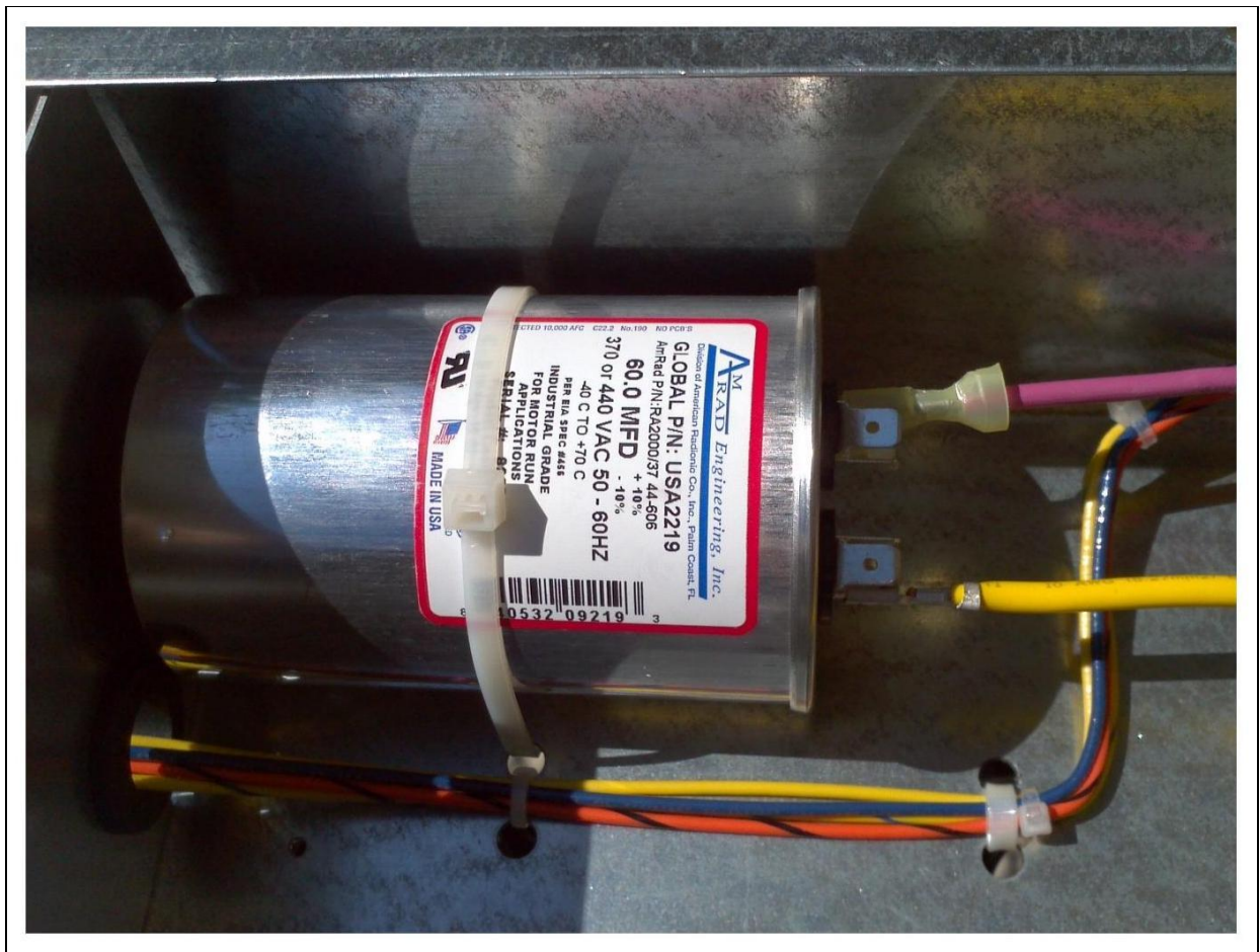
Figure 3. Typical AmRad Run Capacitor Installation
