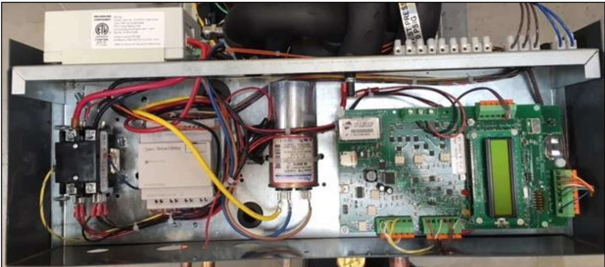
Figure 1 – EDM factory-installed in the Compressor electrical box
